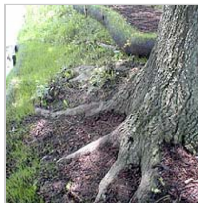
Compost Used as Erosion Deterrent
